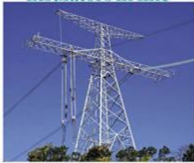
Insulator for EHV transmission line
