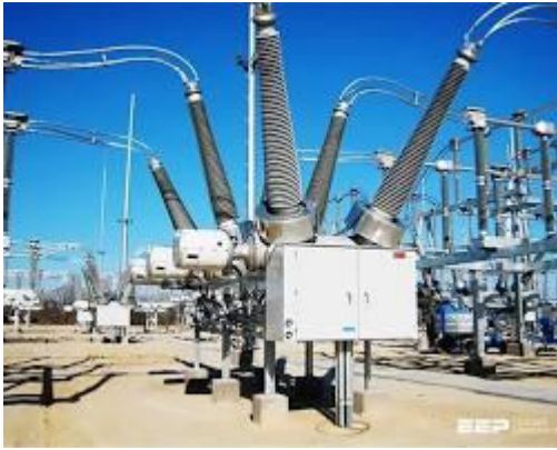
Circuit breaker for EHV transmission line
